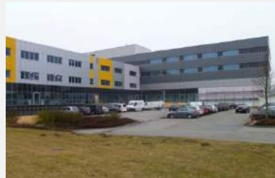
Manufacturing II for final assembly and cleanroom IV expansions.
