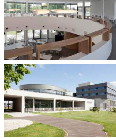
EVG Minis kindergarten / childcare facility and INNside restaurant
